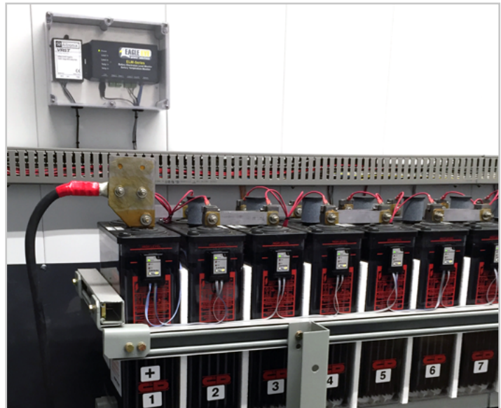
Installation to Battery Cells
