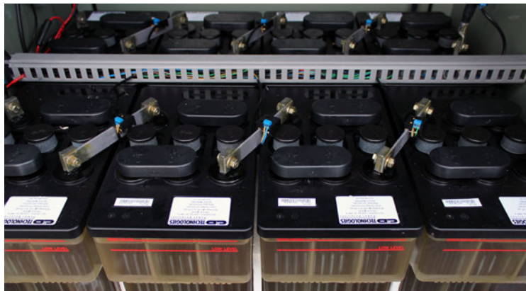
Duct Installation on (8) 6V Jars
