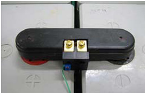
C-Type Clamps Installed to Busbars
