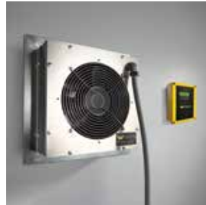
Gas Detection & Ventilation
