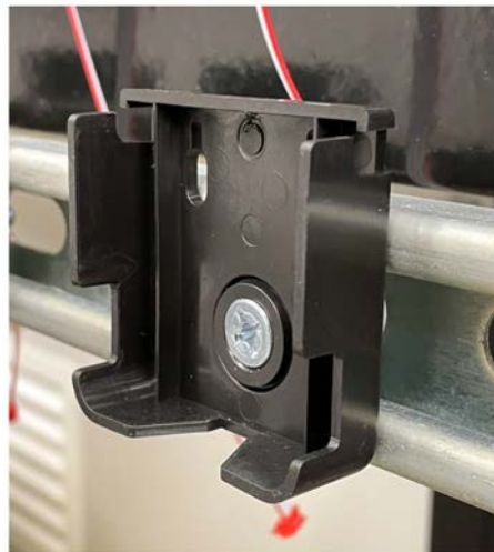
Spring Nut Mounted (preferred)
